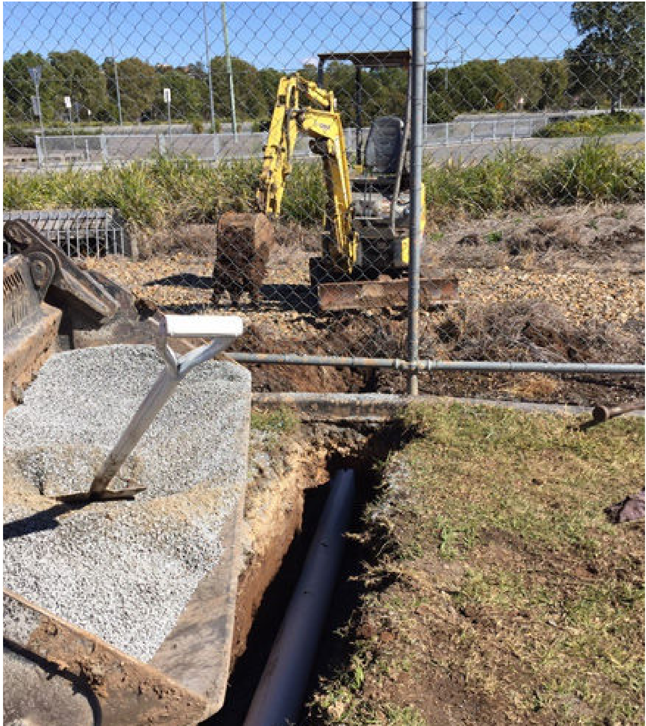
One of the main outlets being trenching in, 200mm PVC stormwater pipe used for outlets
