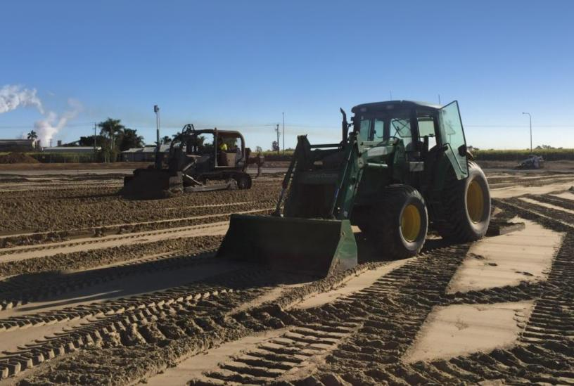
This technique, whilst slightly more time consuming, means that the drainage remains completely intact and compaction and contaminant free once the sand material is pushed out on top.
