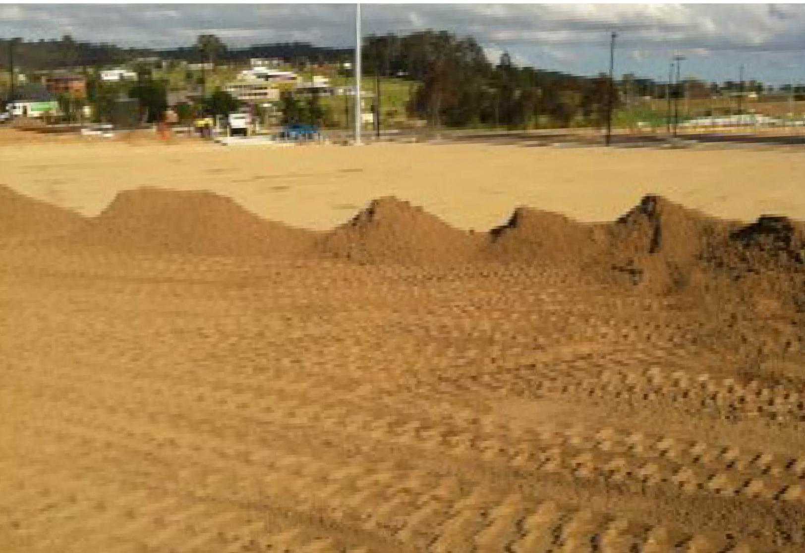
Fertiliser was applied and ready for turf we Installed 10,000 sqm of washed big rolls were installed in 1 mtr x 25 mtr big rolls at rate of a bit over 3000 sqm a day. Once the turf was harvested it was, washed and installed within a 24hr period. It took 3 days to install the main field while all other areas were installed at a rate of 4000 sqm a day.
