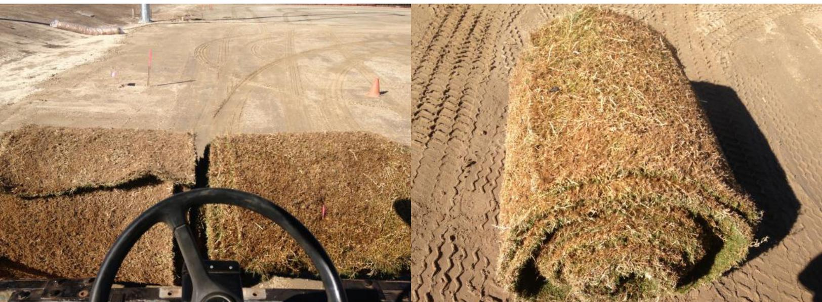
**8** The surrounds; original site soil was used to level and grade the field surrounds, thus saving the cost of importing more material. Some 15,000 sqm of surrounds were levelled and turfed with standard slabs of 'wintergreen' couch. Paths, a car park, fencing and swale drains were built to council specifications and plans to ensure the site was ready for public use.
