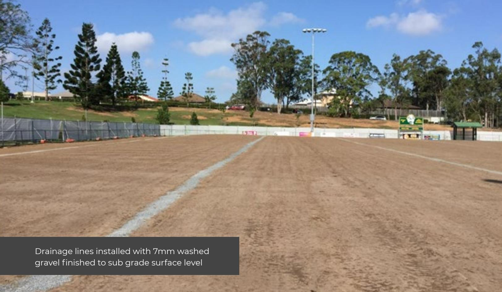
Drainage lines installed with 7mm washed gravel finished to sub grade surface level
