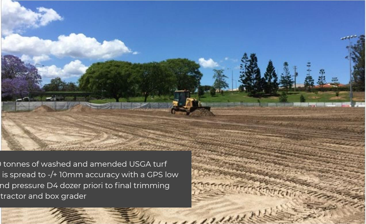
3000 tonnes of washed and amended USGA turf sand is spread to  $\pm 10$ mm accuracy with a GPS low ground pressure D4 dozer prior to final trimming with tractor and box grader
